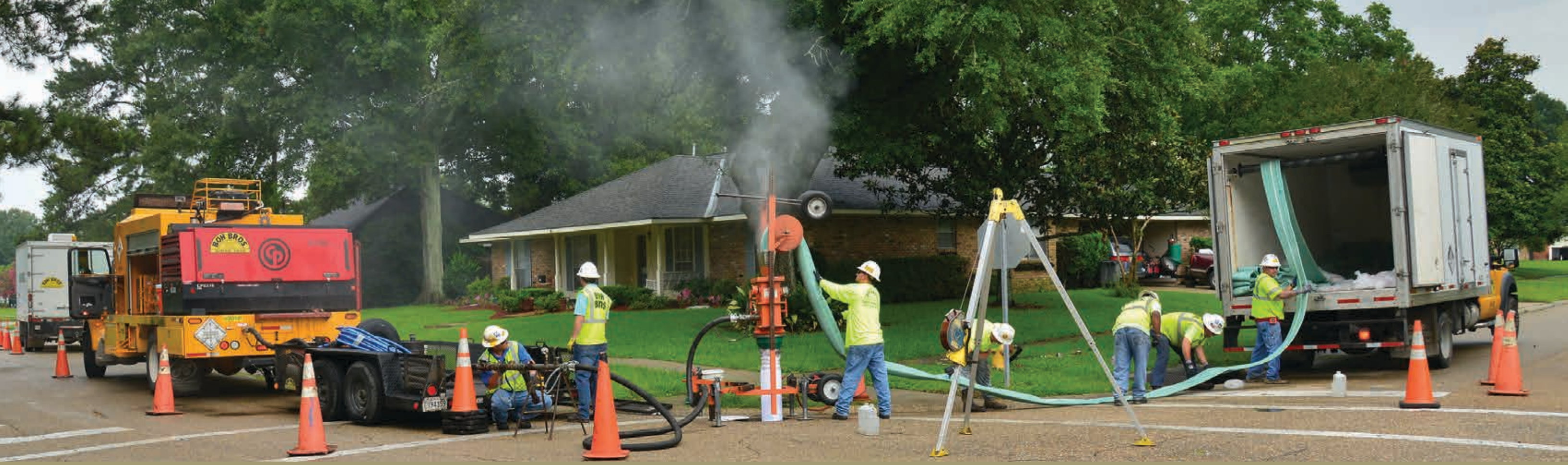
CIPP offers the advantage of providing a continuous pipe from one manhole to another, rather than having joints every 20 or so feet, which are vulnerable to subsidence and tree roots.
