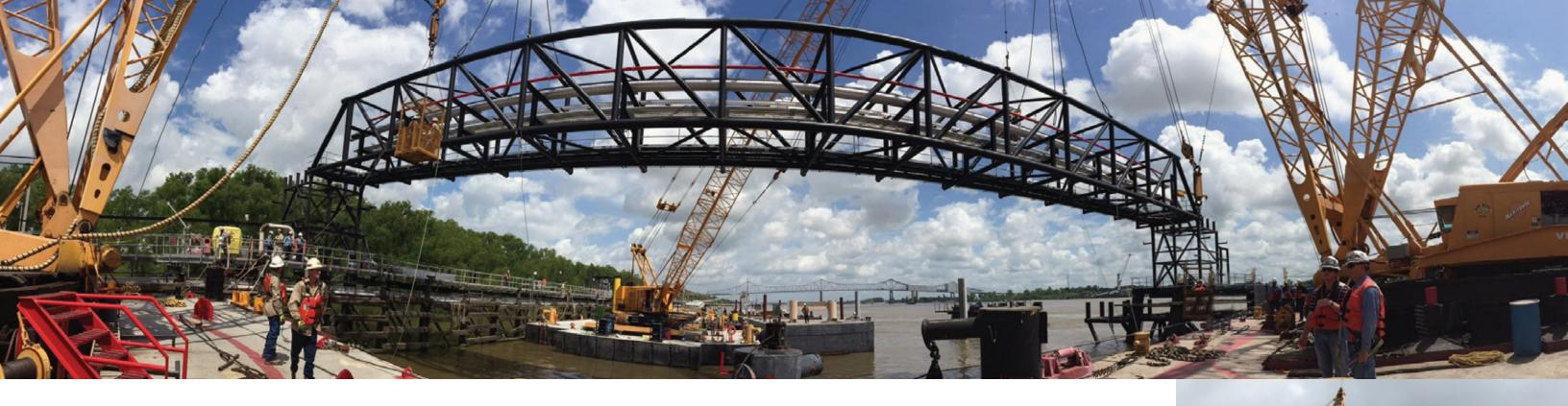
at the Almonaster fabrication yard. Ricky Tamor, fabrication superintendent, said the 206-foot-long bridge was designed with a camber—an upward curvature to compensate for load deflection. "We had to construct the bridge so that it would level itself out when set in place, compensating for the weight of the pipe and other equipment to be installed," Tamor said.
