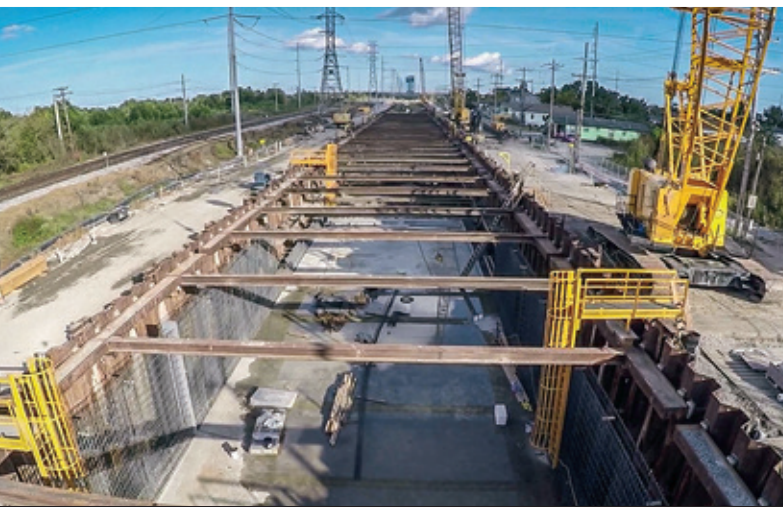
All cofferdam bracing and access ladders on the Florida Ave. Canal project were designed and fabricated in-house. The bolted connections of the bracing struts and wales allow for easy assembly in the field.
