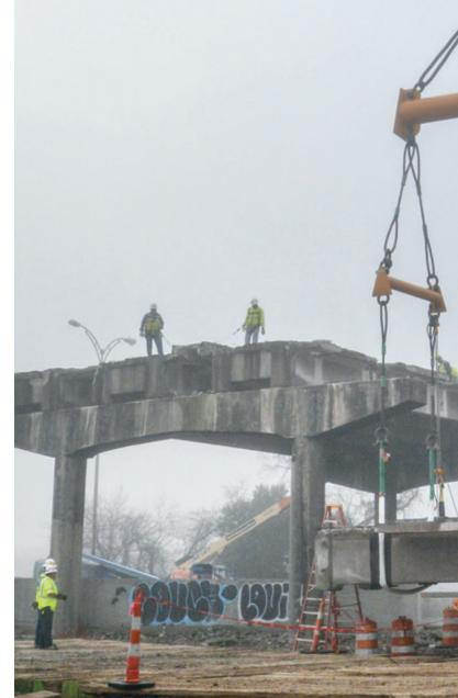
Situated on the east side of New Orleans City Park, the Wisner Boulevard Bridge over I-610 was in decidedly poor shape. The 60-year-old bridge suffered from severe spalling, and reinforcing steel visibly protruded from the concrete. *(continued next page)*
