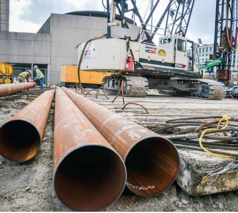
two existing buildings with limited space in an area the size of a small office. To compensate, the Boh crew utilized a forklift and hammer to drive the pile in pieces. Since a load test would have been difficult in such a limited space, the testing company relied solely upon a PDA to measure bearing capacity. Ultimately, the pipe piles will support an animal transport bridge connecting two oncampus structures, and the timber piles will support a large generator building.
