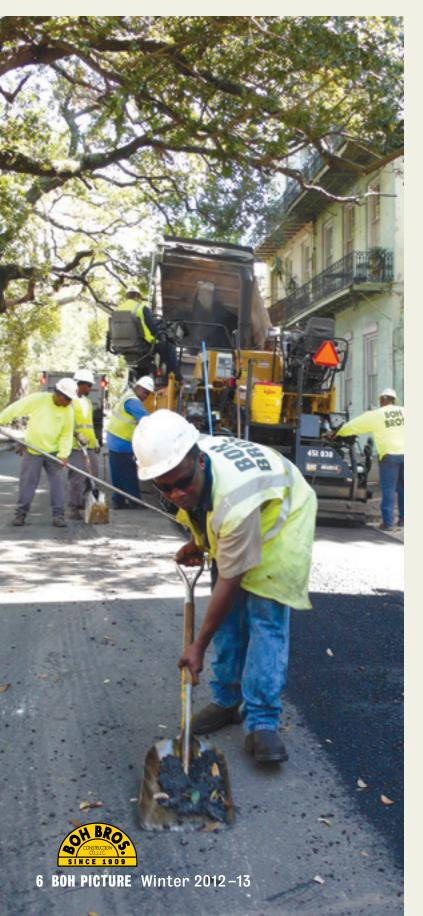
started on Burgundy Street and worked in half mile sections as traffic was rerouted," Alexander said. "After milling a section we would follow sequentially with the overlaying, so we had a
